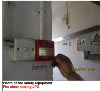
Photo of fire safety equipment Fire alarm flashing when tested.JPG
